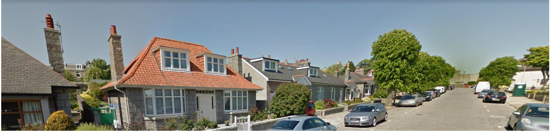
5 - Red tile roof at 28 Craigie Park
