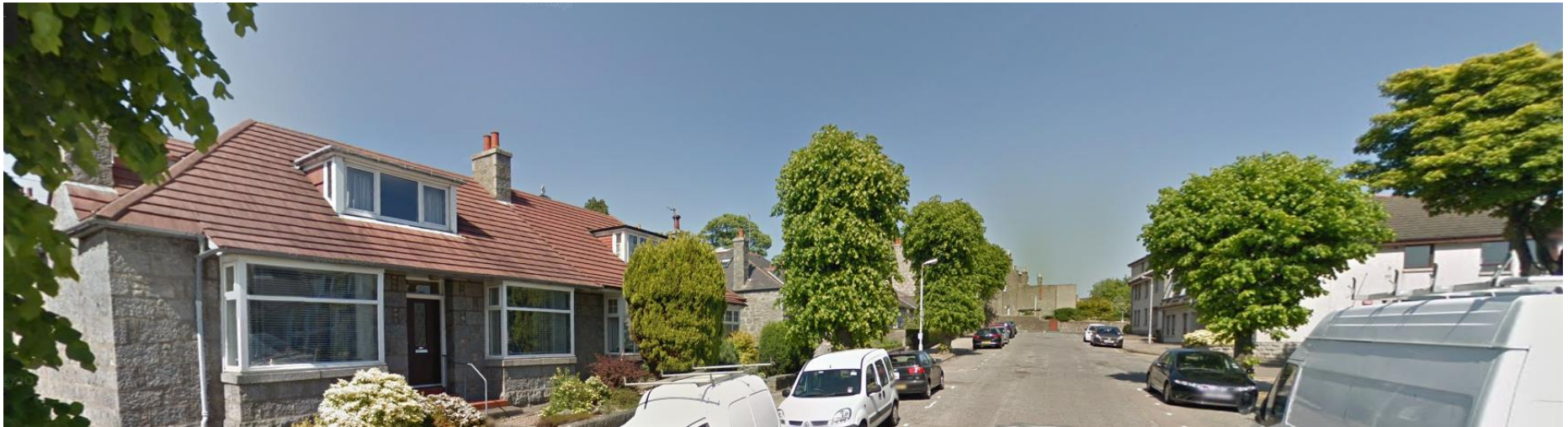
6 - Red tile roof at 16/18 Craigie Park
